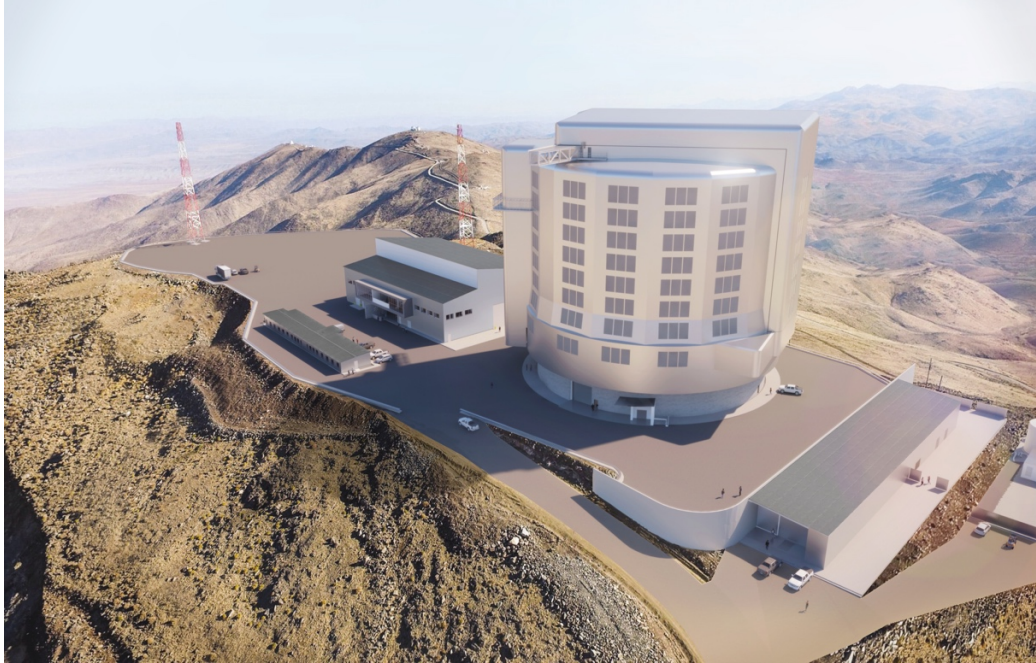
Figure 20. A rendering of the enclosure and facilities buildings on the summit of Cerro Las Campanas on property owned by the Carnegie Institution for Science. The summit site includes (from left to right): summit construction offices; summit support building, housing the primary mirror cleaning and re-coating equipment; enclosure; and summit utility building (SUB). The SUB supplies and distributes the telescope utilities, including electrical power, liquid coolants, and gas refrigerants (compressed CO 2 and compressed helium). The SUB is connected to the enclosure through the summit utility tunnel (not shown). Additional facilities will include the shop, warehouse, and utility yard at support site #1.
