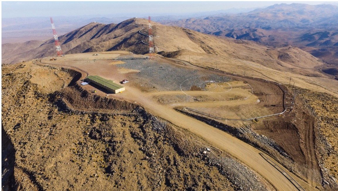
Figure 13. View of the summit site mesa looking North toward the Las Campanas Observatory. Construction offices are seen on the left. Concentric white circles (enclosure and pier concrete ring wall diameters) indicate the future location of the GMT.
