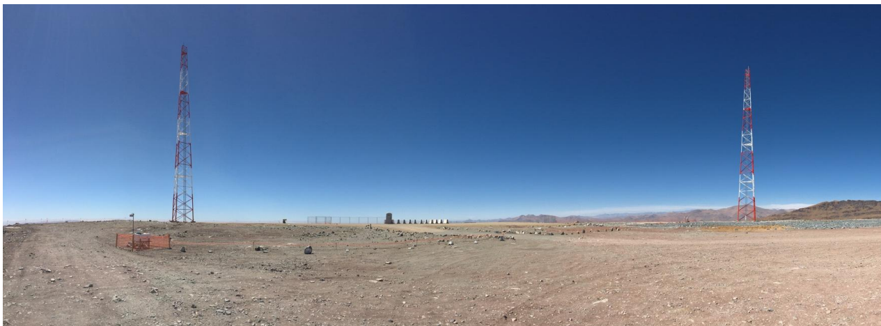
Figure 9. Instrumentation towers at the GMT site. These host the scintillometer that is being used to characterize the ground-layer turbulence, weather stations, and cameras that will monitor and record construction.
